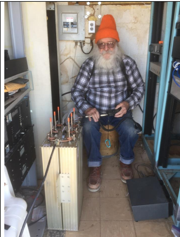
Dennis Prepares for the Duplexer Install
